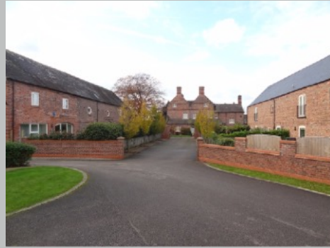
Plate 34. Side (E) elevation of Kinderton Hall and barns of differing ages
