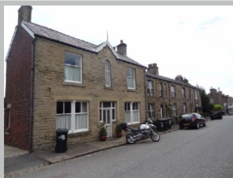
Plate 10. Terrace on Shrigley Road in front of part of site
