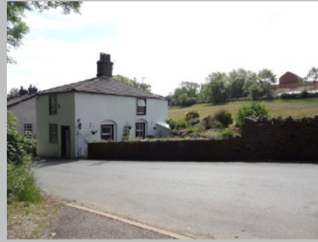
Plate 23. White Cottage with site behind
