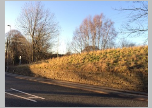
Plate 8. Stone wall at W end of site frontage
