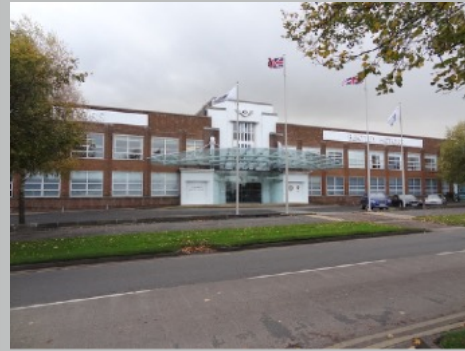
Plate 14. Bentley's Showroom Building
