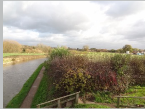
Plate 30. View E along N boundary of E part of site from bridge, with canal, towpath and site elevated on embankment and behind hedge in winter
