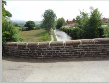
Plate 22. View over site and canal from Bridge 26
