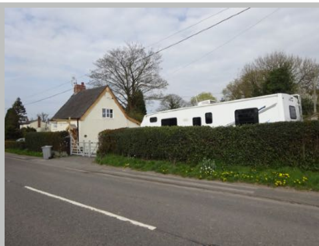
Plate 54. RH (SE) gable of Holly Cottage
