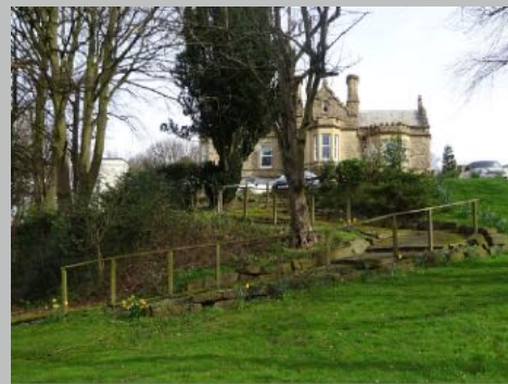
Plate 16. View of Hollin Hall Hotel from site
