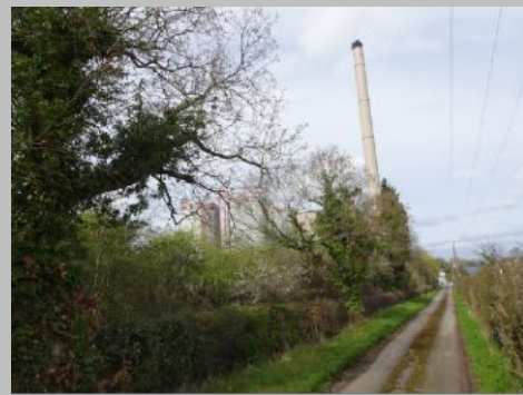
Plate 41. Chimney and tanks inside E boundary
