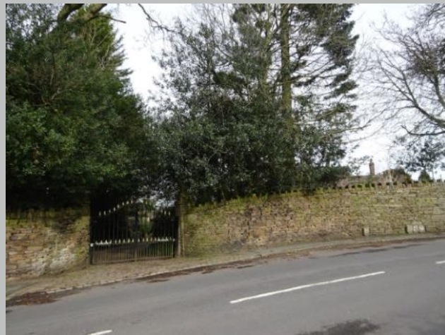
Plate 4. Hollin Old Hall (roof of) and entrance to it from NW edge of site
